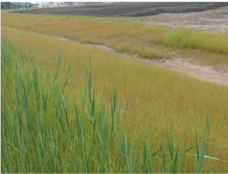
Photograph 4: View of the stormwater management swale surrounding the western, southern, and eastern portions of the ash impoundment area on the subject property.
