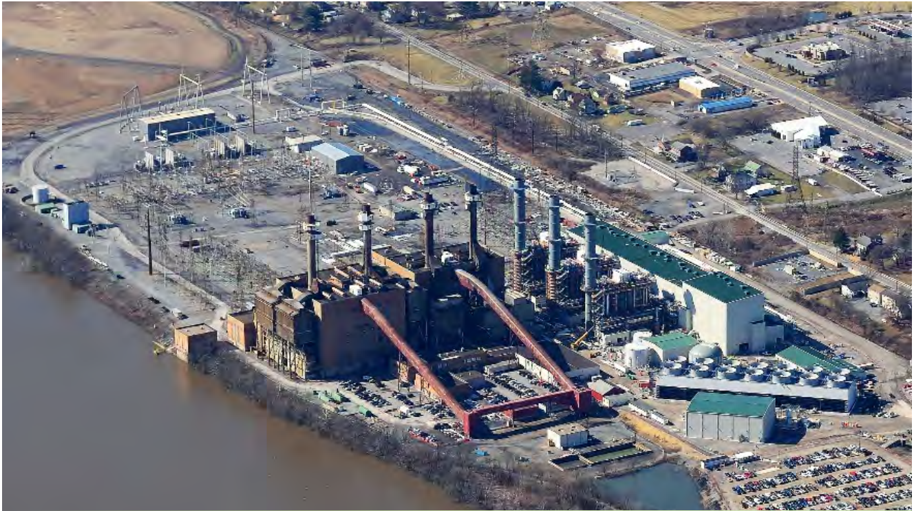
Sunbury Generation Power Plant
