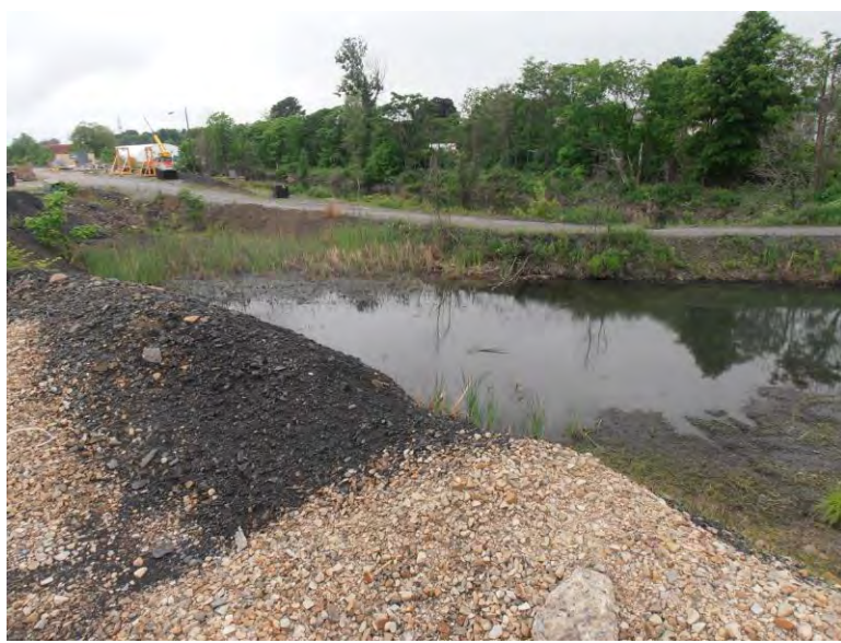
Photograph 19: View of one of the western stormwater retention ponds on the former coal storage area on the subject property. Coal residue seen in and around the pond.
